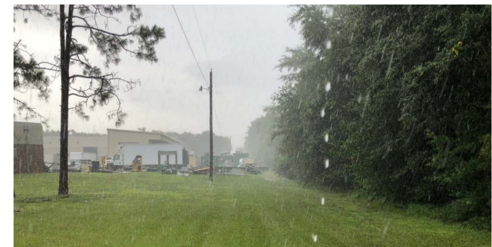
Utility corridor adjacent to the Florida Turnpike (right) and behind the Gateway High School (left).
