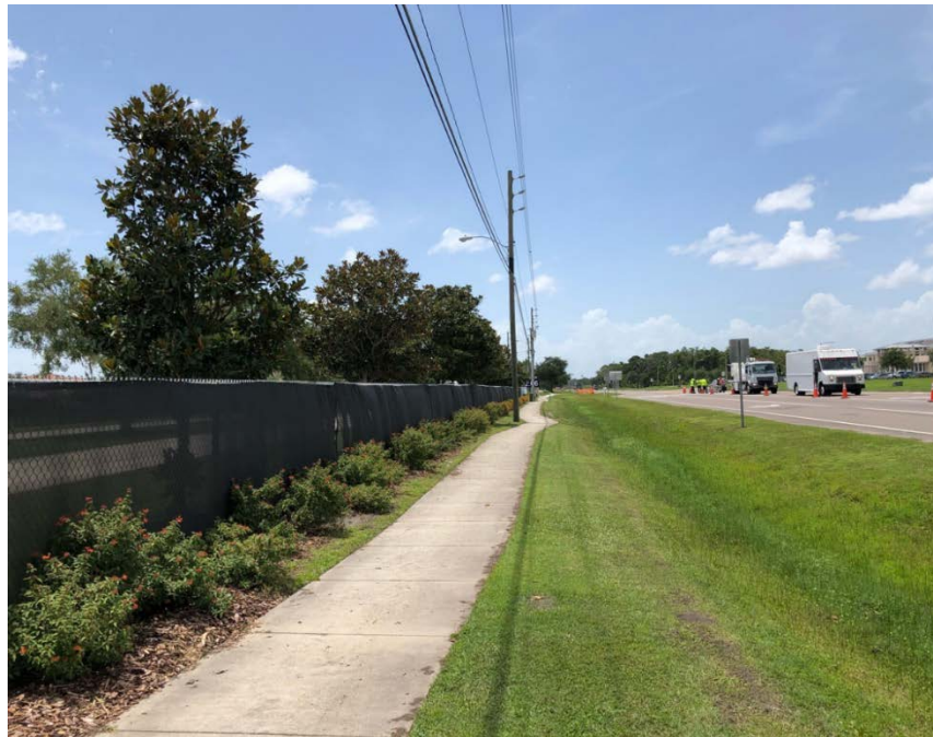
Typical south side sidewalk. Significant right-of-way near Austin Tindall Park. Possibly extend sidewalk and modify swale.
