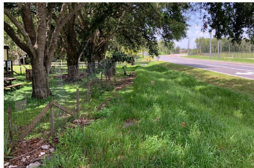
South side of Boggy Creek Road with open drainage and lack of sidewalk adjacent to private property.
