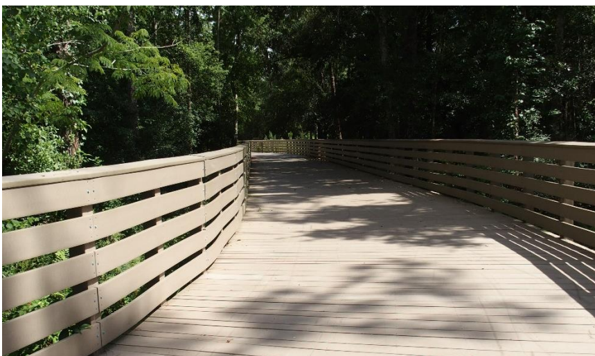
Shingle Creek Trail boardwalk – south of US 192
