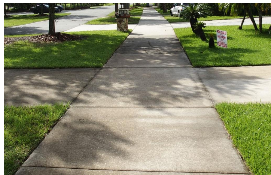
Existing level driveway crossing on the Neptune Road cul-de-sac.
