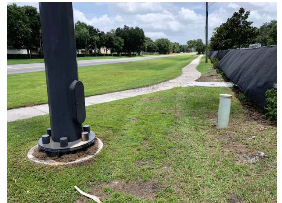
5' existing sidewalk on south side of Boggy Creek Road in front of Austin Tindall Park.
