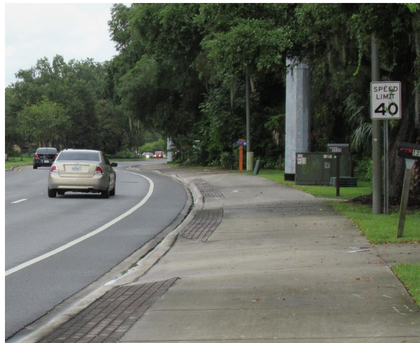
Typical driveway apron sloping across the trail on Neptune Road northwest of the Bill Johnston Rest Area.
