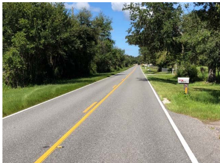
Facing west along Reeves Road showing the typical existing roadway conditions along Segment 1.
