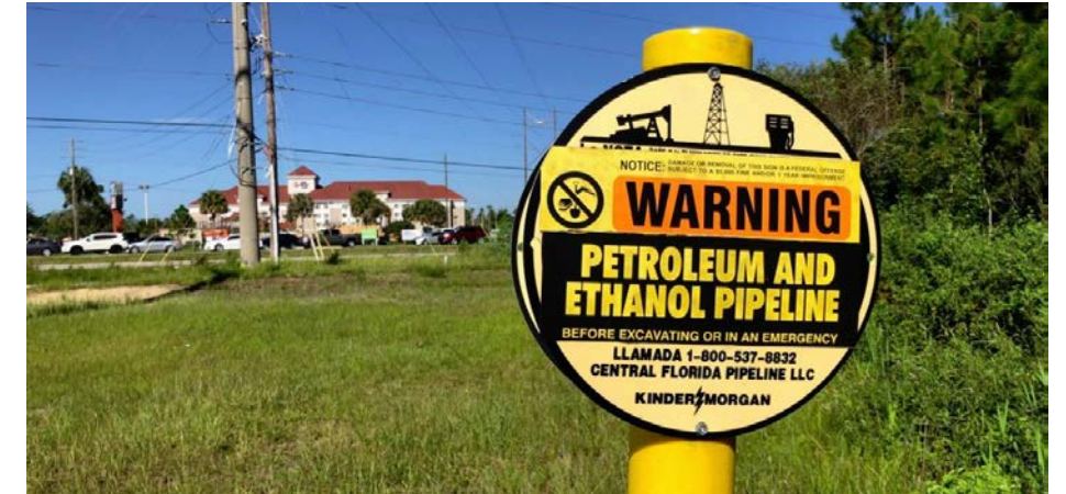
Central Florida Pipeline utility marker in easement near SR 535.
