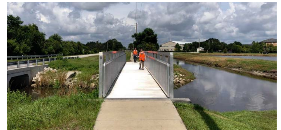
Existing 6' metal modular bridge over the drainage canal in Segment 1.
