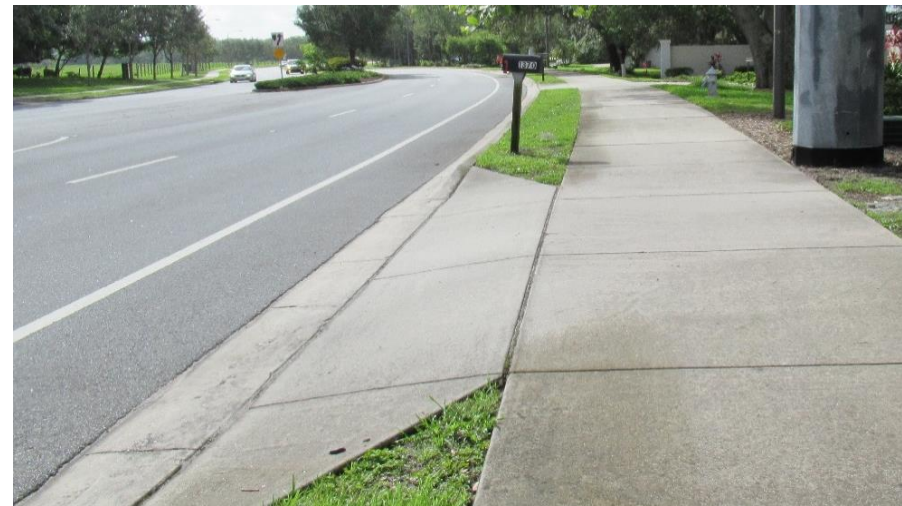
Example of an existing driveway apron on Neptune Road that slopes down only in the parkway strip.
