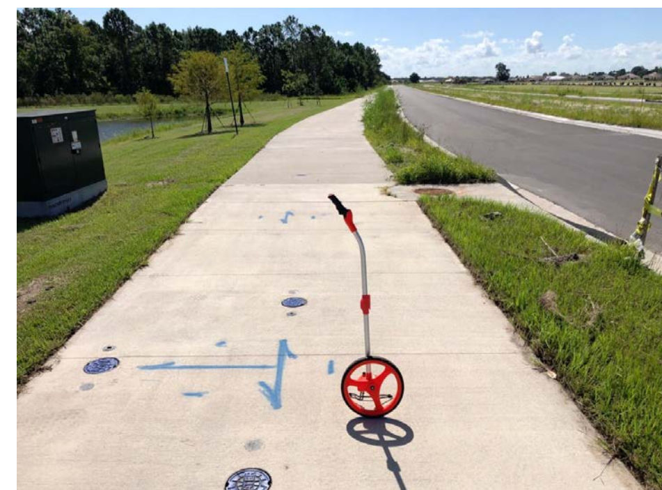
An 10-foot-wide existing sidewalk along the north side of Interior Street east of Pleasant Hill Road.
