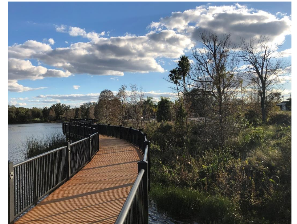
Example boardwalk style bridge with classic black finishes and natural littoral plantings adjacent to US17-92 in Casselberry, Florida.
