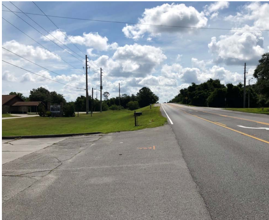
North side of Partin Settlement Road facing east. Utility placement approximates future bridge width.
