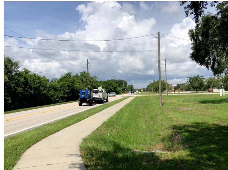
The westbound approach to the future Partin Settlement Road/Cross Prairie Parkway intersection. Existing sidewalk is currently in the future turn lane.
