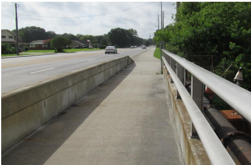
Existing Neptune Road bridge and 'back of curb' trail facing east.
