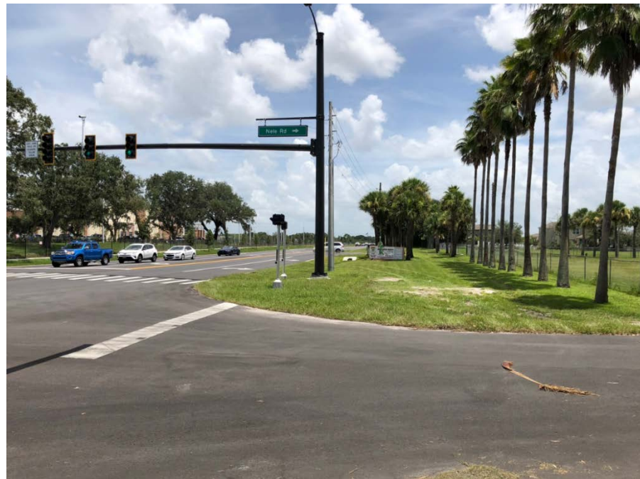
New signalized intersection for Tohopekaliga High School would require pedestrian crossings for the trail.
