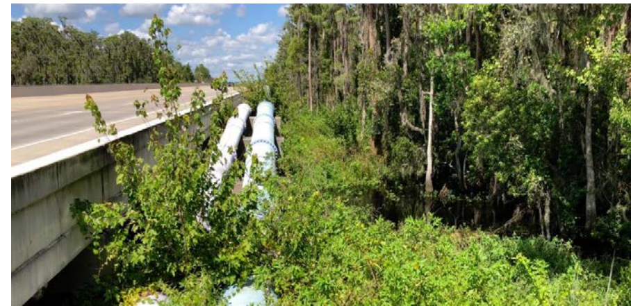
Proposed trail bridge designed separately would cross Shingle Creek on the north side of Osceola Parkway.
