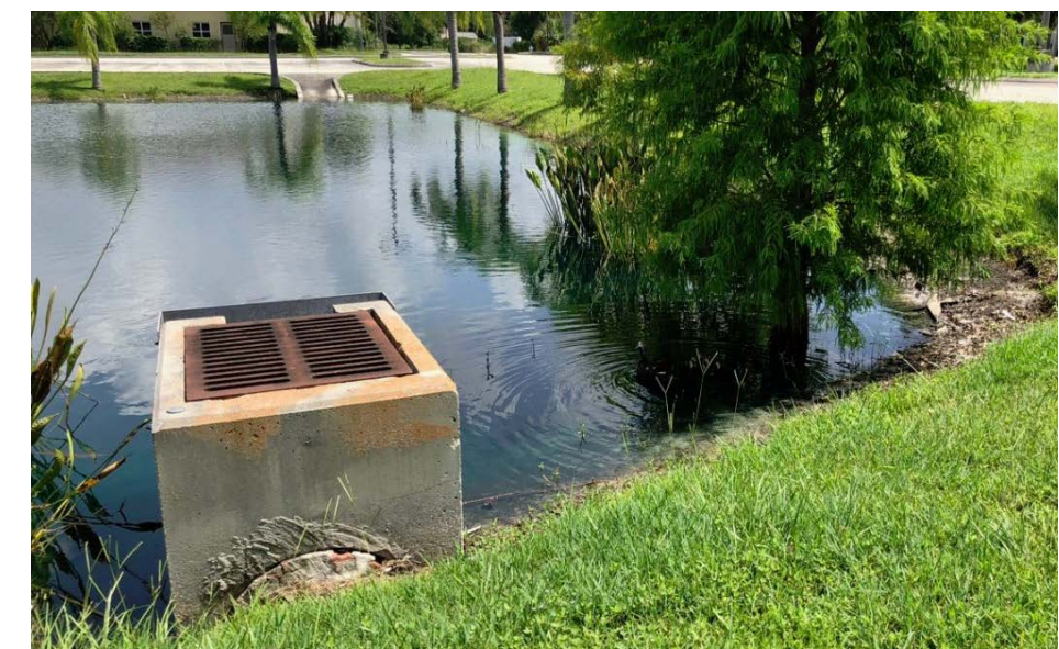
Drainage retention area in front of ice rink on the north side of Partin Settlement Road. Possible rest area location along trail.
