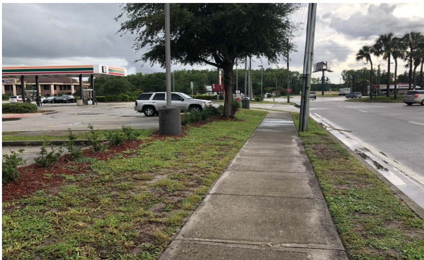
Right-of-way in front of private property (left) on the southeast side of Bill Beck Boulevard.
