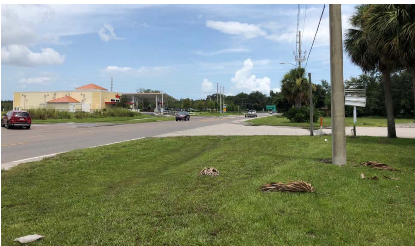
Typical south side of Boggy Creek Road approaching Narcoossee Road. Significant right-of-way with no existing sidewalk.
