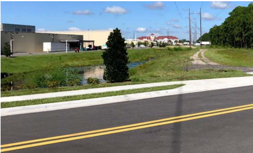
Poinciana Boulevard extension. Existing access road for utilities behind shopping center.
