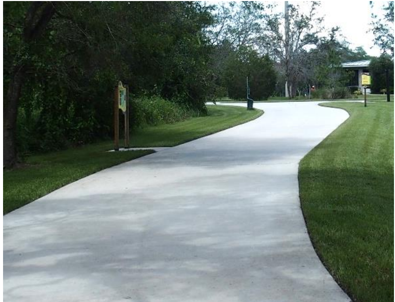
SHINGLE CREEK TRAIL HORIZONTAL CLEARANCE
