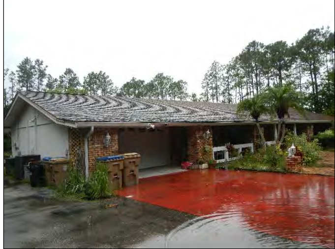
Figure 18. Resource 8OS02921, facing southwest.
