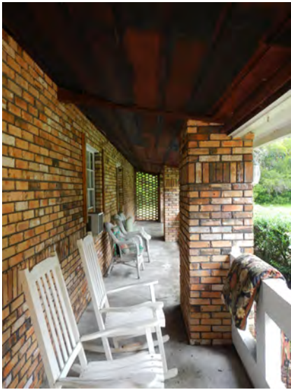
8OS02921_a Facing West
