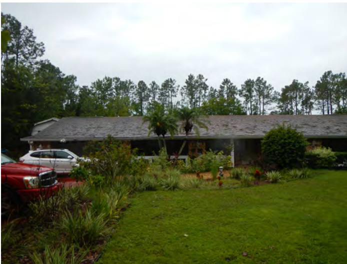
8OS02921_e Facing South
