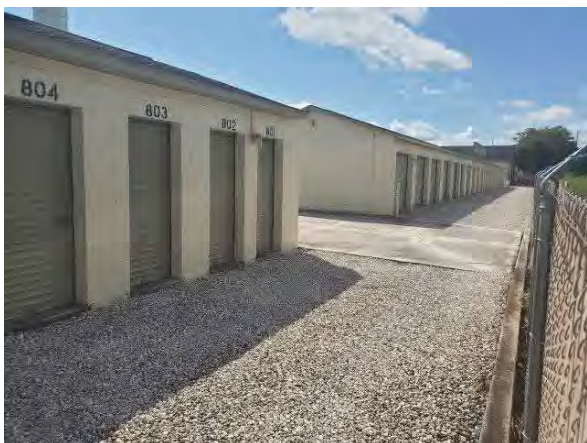
Photo #65 Central Mini-Storage
