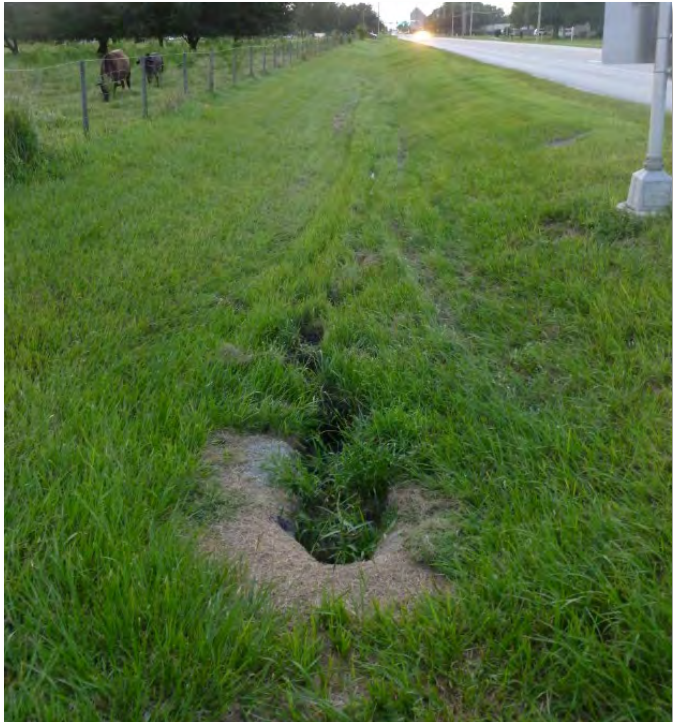
Figure 9: Typical upland-cut ditch, adjacent to Pond Site 8A(1)
