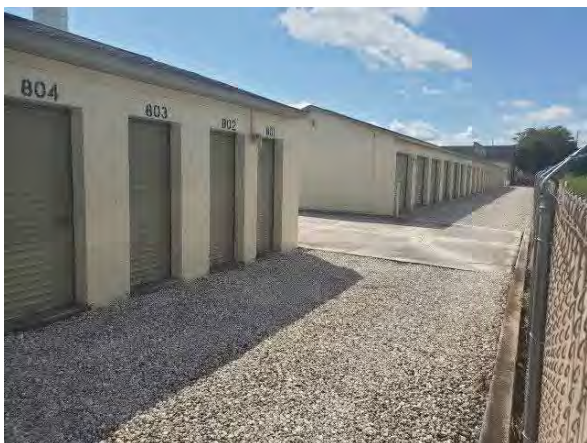
Photo #65 Central Mini-Storage
