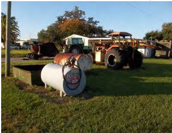
Photo #129 Pond 5(3) Diesel and Waste Oil aboveground storage tank (AST) with minor staining of soils.
