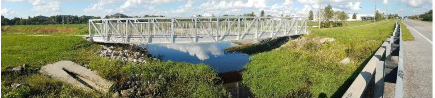
Pedestrian bridge. Facing north from Partin Settlement Road.
