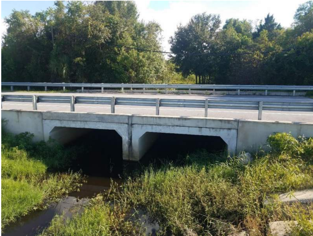
Partin Settlement Road box culverts. Facing south.
