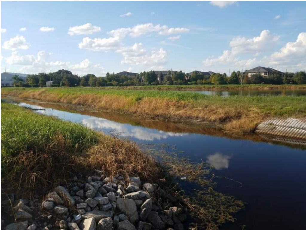
Fennel Slough canal northwest of box culverts.
