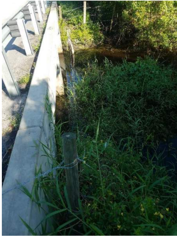
Downstream (southern) end of existing box culverts.
