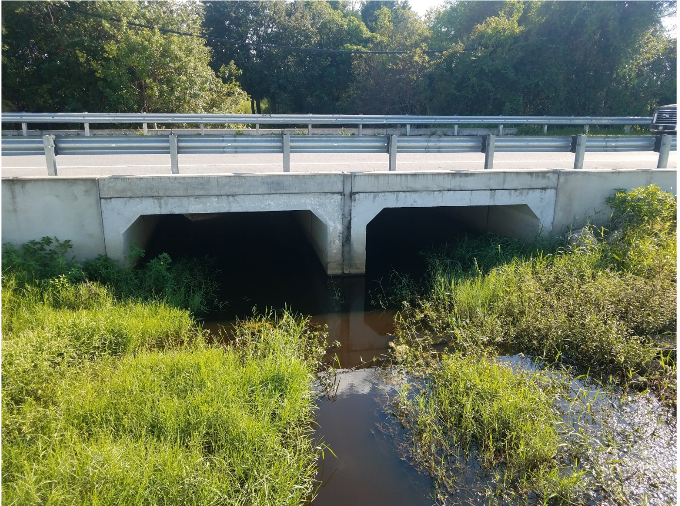
Figure 1. North side of box-culvert facing south and downstream
