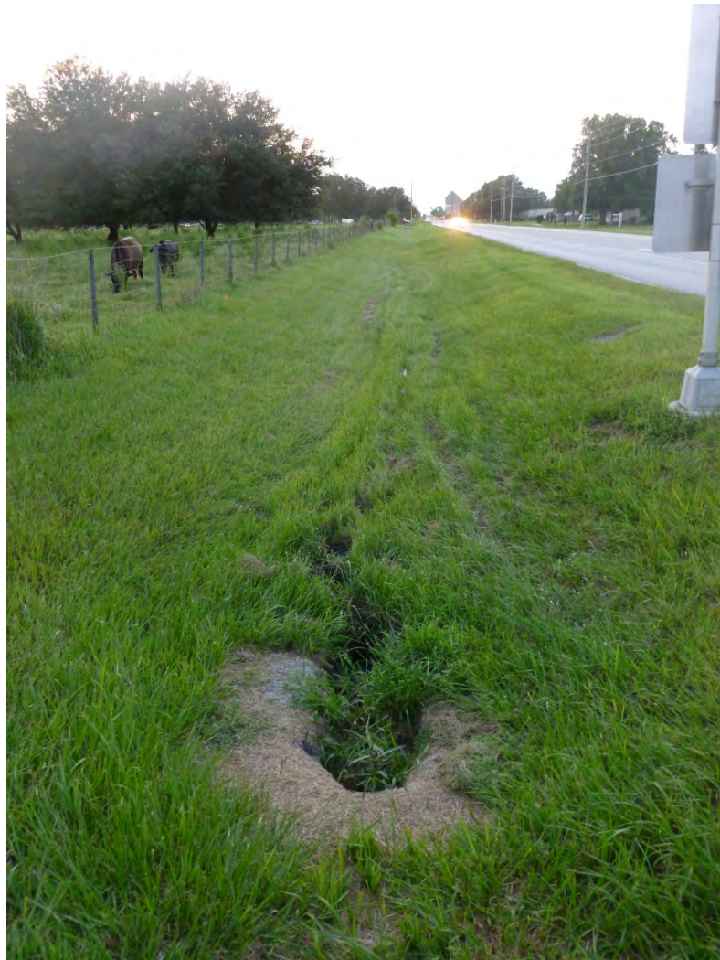
Photo 1: Typical upland-cut ditch, adjacent to Pond Site 8A(1)
