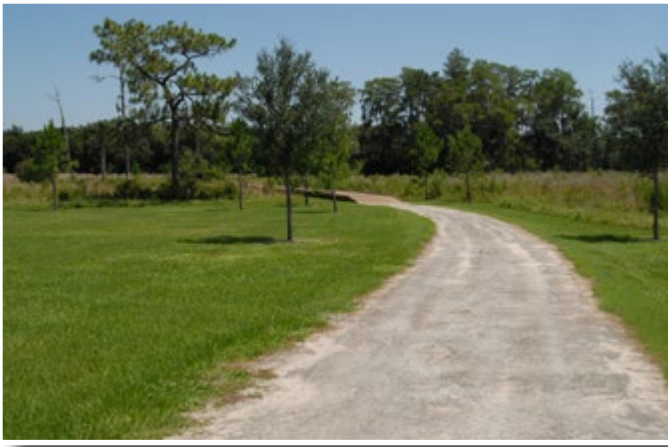
Typical Soil Cement Trail
