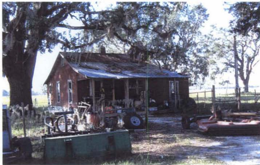
8OS2392, SOUTH AND EAST FACADES
