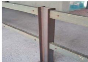
Steel beam posts + wooden rails
