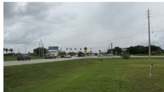
Existing rural highway section
