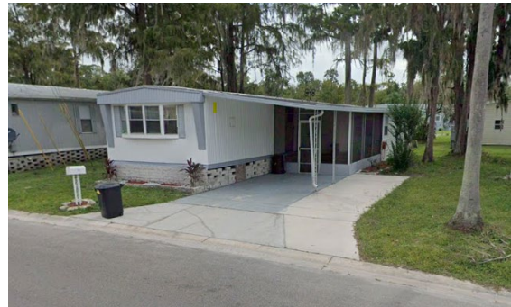
Structure elevated 1-2 feet; guttering draining to driveway and street
