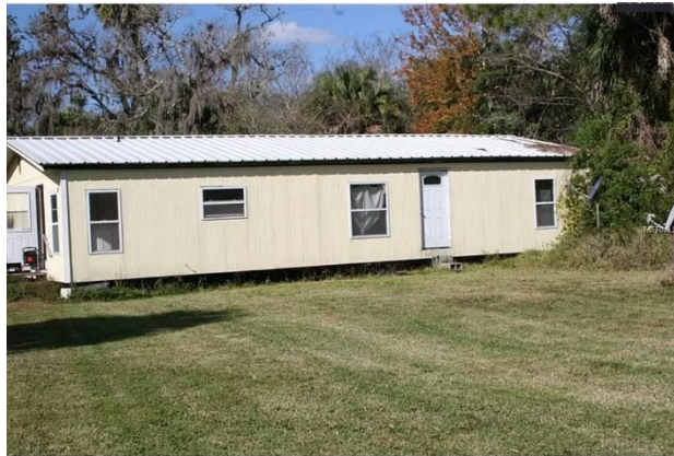
Manufactured home raised on block foundation
