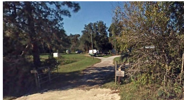
Drainage ditch and culvert under driveway
