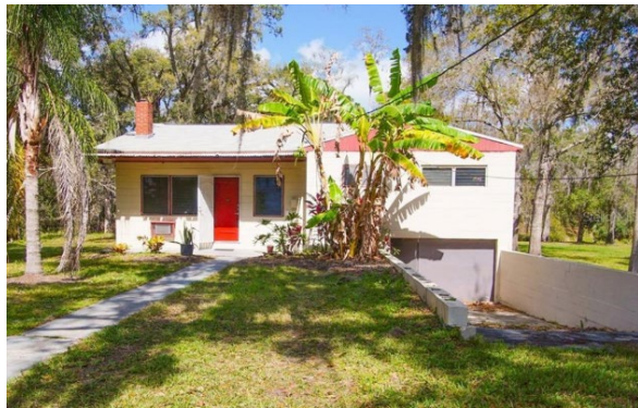
Residential structure with below-grade driveway/garage/storage
