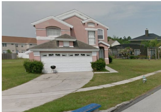
Stormwater inlet in front of house
