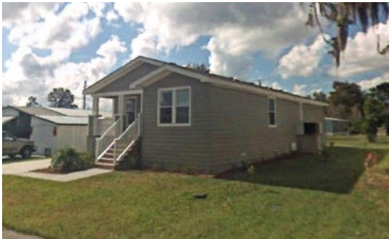
Structure and HVAC elevated above BFE
