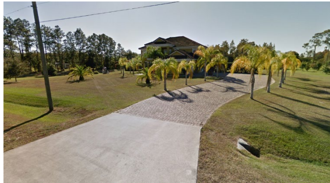
Drainage ditch and culvert along road and under driveway
